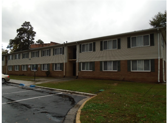
Subject's exterior and typical surface parking
