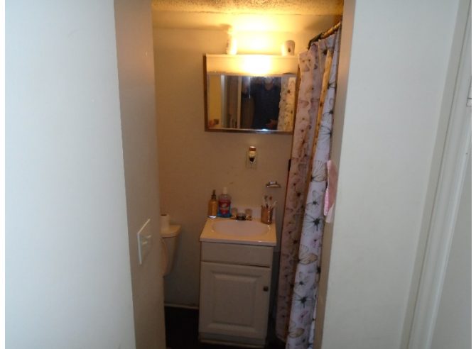
Typical bathroom (view one of two)
